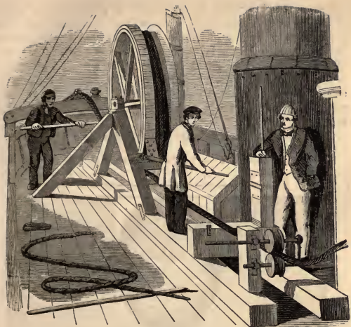
Fig. 34.—LAYING THE CABLE FROM THE DECK OF THE SHIP.
